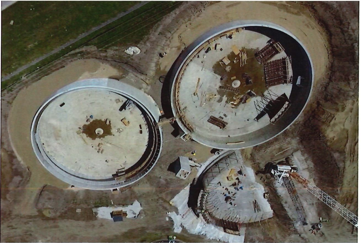
Aerial View of Clarifiers March 28, 2024
